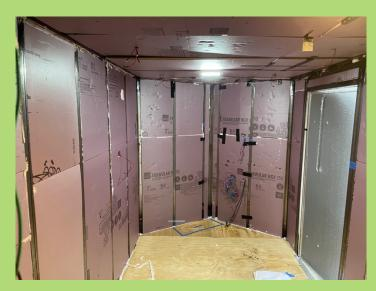
**Cracks:** It is inevitable that the boards won't fill every spot perfectly. This is where I used the small cans of foam insulation. These are commonly used around windows but I also found they work great around cracks and other areas where the foam board didn't fit in too well. Additionally, this prevents movement when you are on bumpy back roads on an adventure.
