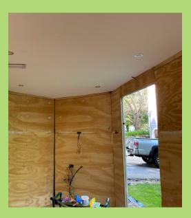
Method: There are a lot of unique different cuts and holes that need to be made. Don't hold yourself to one tool or method. I ended up using a jigsaw, table saw, circular saw, and miter saw all in this step. Having tool proficiency and experience makes this step a lot easier and less tedious.
