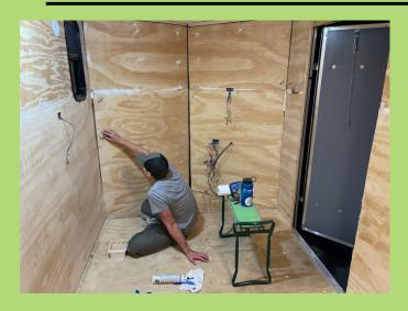
**Prep:** Since I reused the plywood there was a lot of prep needed. I used a spackle/wood filler mix to fill all the screw wholes and other crack. I also used caulking to fill larger gaps. It was important to remember that I was going to have trim to cover up a lot of imperfections as well. The final step was sanding everything to be smooth for paint.
