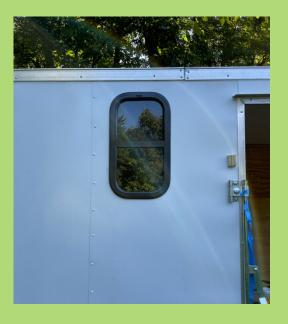
Install: This is another step where a helper is needed. Someone will need to push the window in form the outside while you add the inner part, creating a pinch. You will want silicone inside of the connection, as well as surrounding the whole window. You will also want to make sure that the window is oriented correctly. You want the bottom half to slide up. I suggest having at least 2 windows. It allows there to be a cross breeze, as well as lots of natural light.
