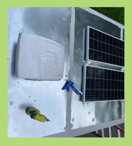
Sealing: The most important part of any hole or alteration is sealing it back up. There is no such thing as 100 % silicone. Put it in the hole before you put a screw, put it on the screw, put it on top, put it on the inside. A small leak down the road can ruin everything that you have built.
